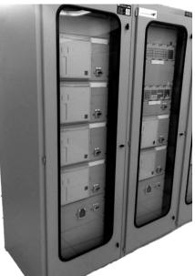
Fig. 2 – Method of MPD Installation into Cabinets in Use Today.
