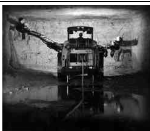
Figure 1: Drill Jumbo at work underground (photo courtesy of Atlas Copco).
