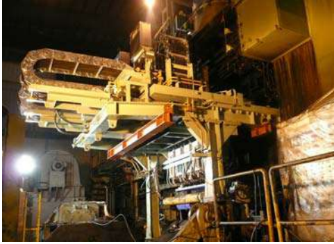
Figure 11. Zoom device in erection
