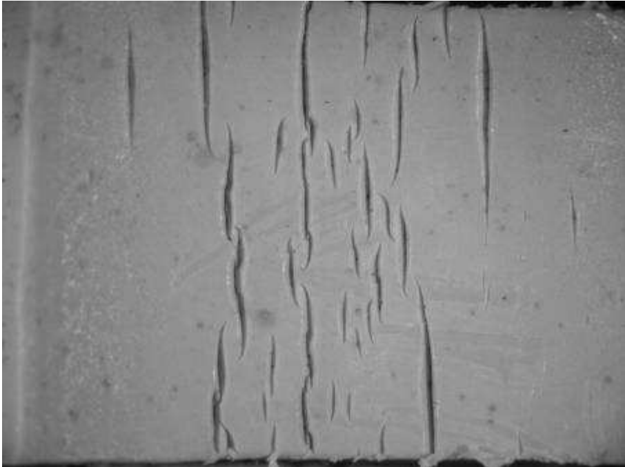
Figure 5. A close up of the surface with the cracks.
